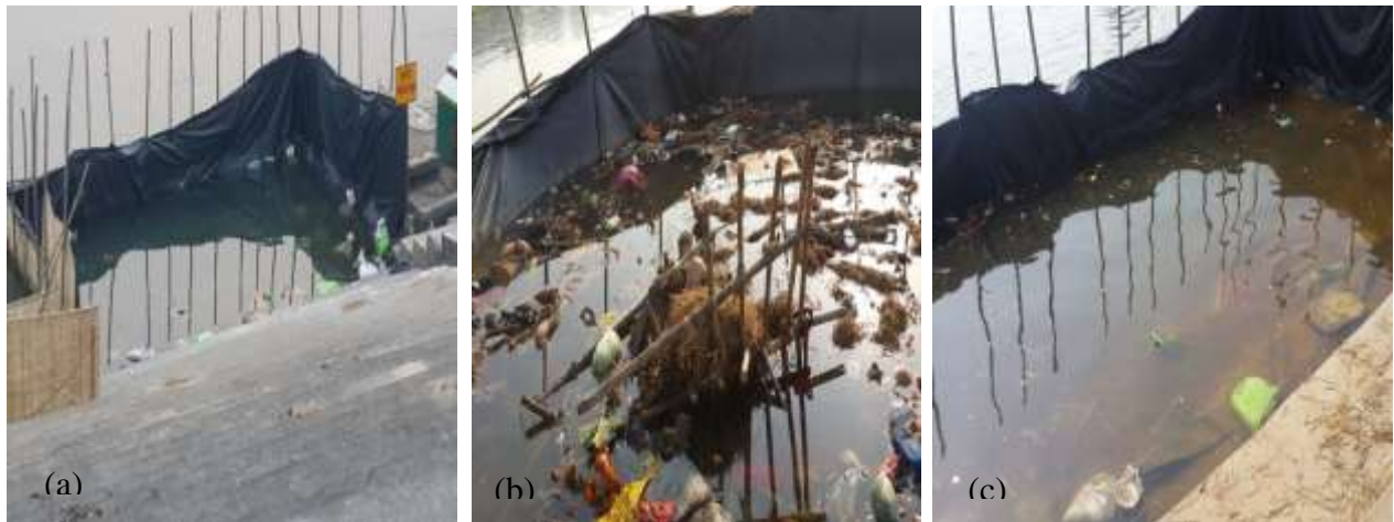
Temporary Idol immersion pond created by barricading a portion of the Mahanadi river on its bank at Balibandha ghat , Sambalpur
