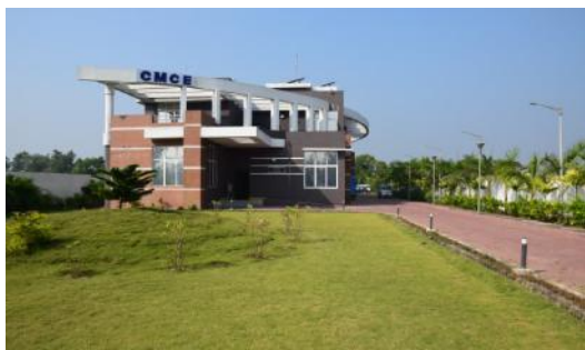
CMCE Building in Paradeep
