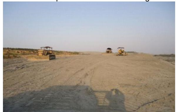
Ash disposal site
