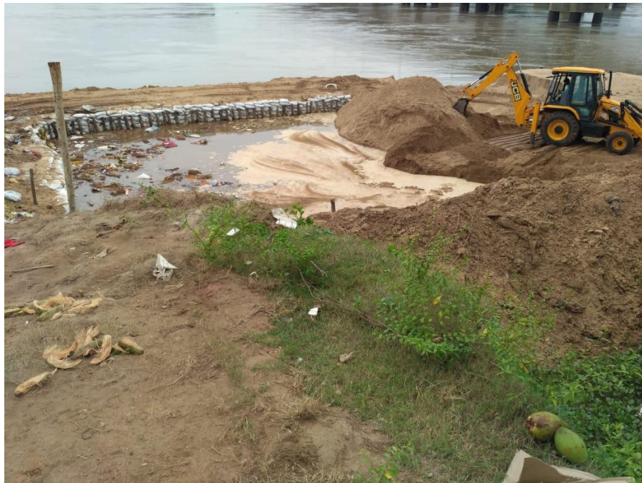
Fig. 6 Condition of temporary immersion ponds after 48 hours of immersion
