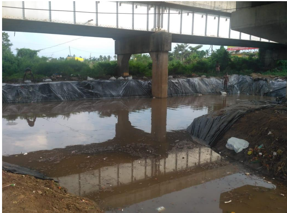
Fig. 5 Condition of temporary immersion ponds after 48 hours of immersion
