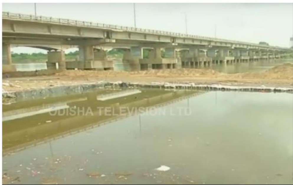
Fig. 2 Temporary immersion pond on the bank of Kuakhai river along Bhubaneswar
