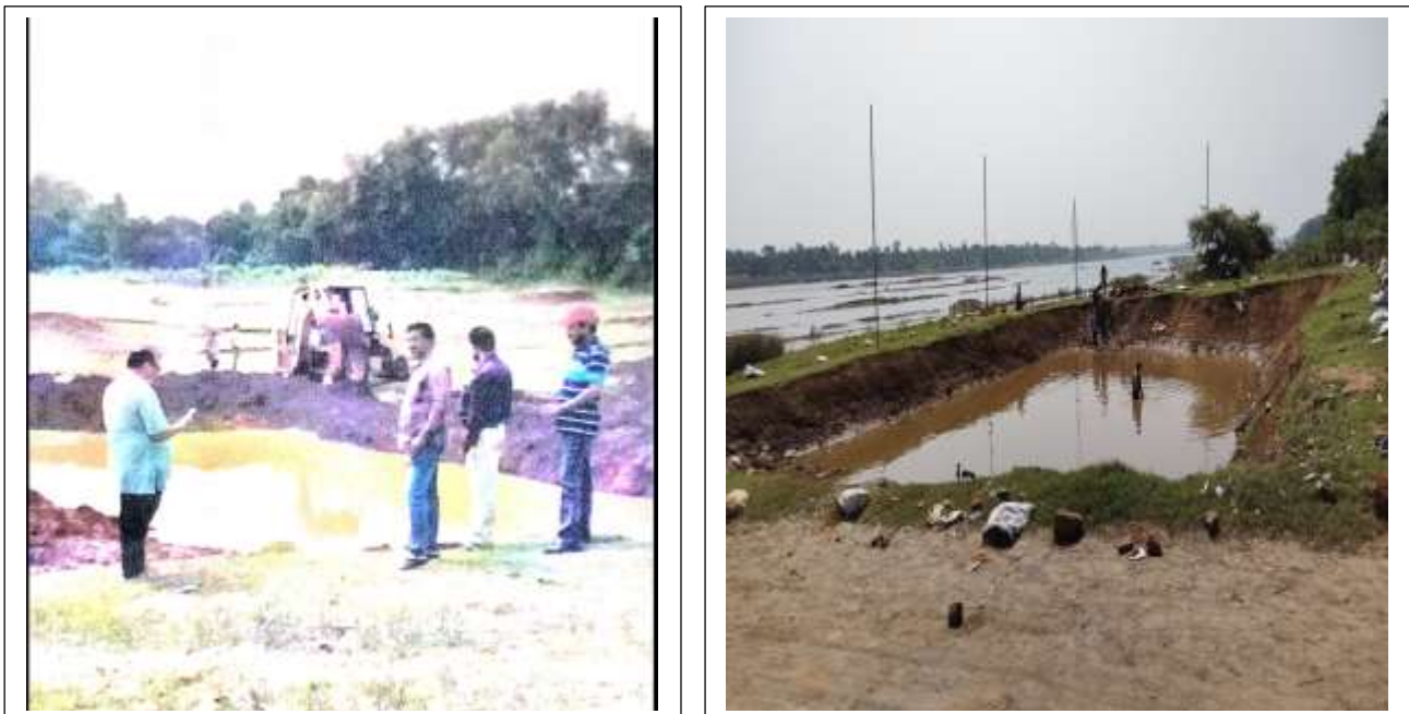
Fig. 2 Construction of temporary idol immersion pond on the bank of river
