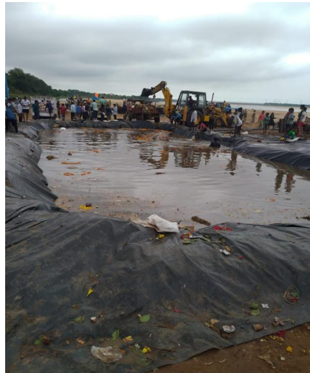
Fig.9 Removal of immersion left overs by Scavangers
