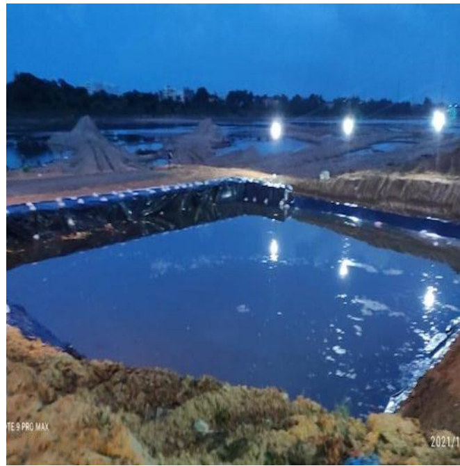
Fig.4 Lining of temporary idol immersion ponds with synthetic liner
