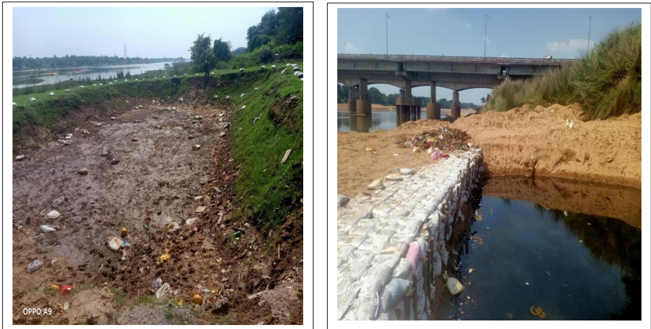
Fig. 3 Construction of temporary idol immersion pond on the bank of river
