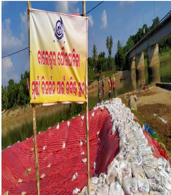
Fig.4 Lining of temporary idol immersion ponds with synthetic liner
