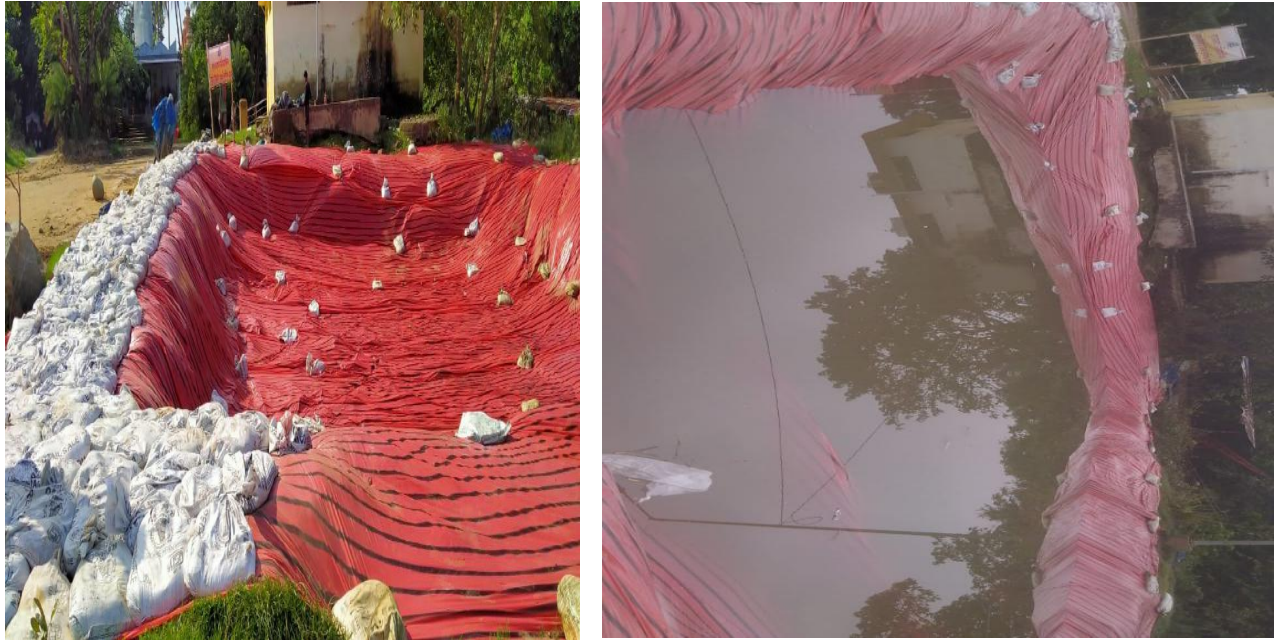
Fig.4 Lining of temporary idol immersion ponds with synthetic liner
