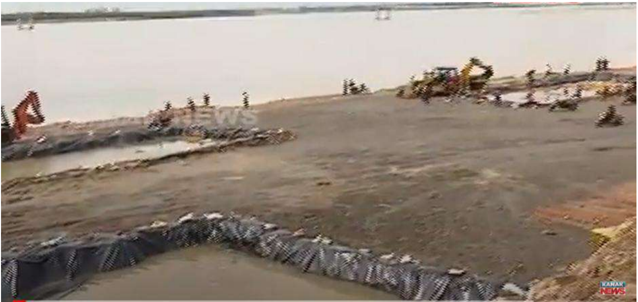
Fig. 3 Construction of temporary idol immersion ponds on the bank of Kathajodi river at Devigada, Cuttack
