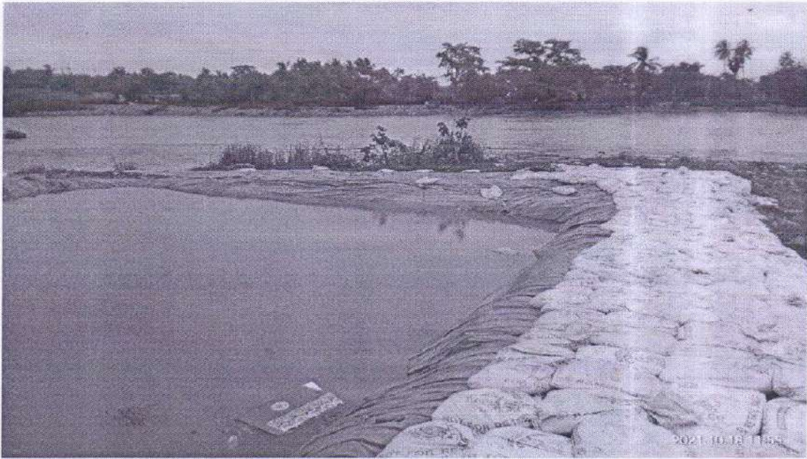
Artificial idol immersion Pond constructed by Balasore Municipality
