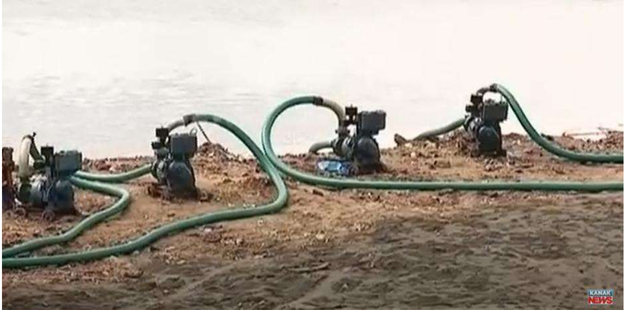
Fig.4 Filling of temporary immersion ponds with River water
