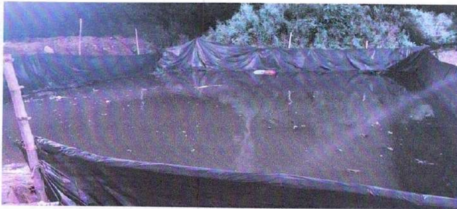
Idol Immersion Pond with synthetic liner provided by Balangir Municipality
