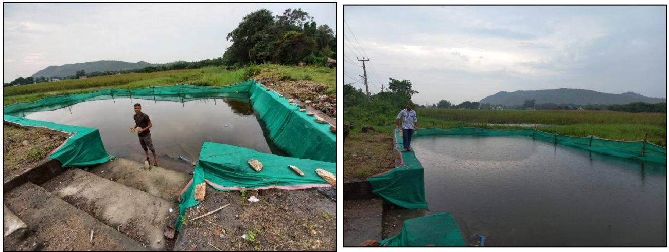
Fig. 5 Construction of Temporary immersion ponds in Cuttack
