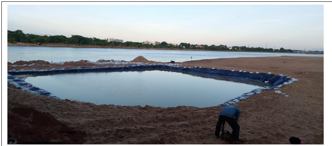
Fig. 4 Construction of temporary idol immersion pond on the bank of Kuakhai river in Bhubaneswar
