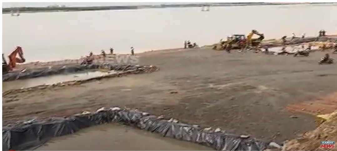
Fig. 5 Construction of temporary idol immersion pond on the bank of Kathajodi river in Cuttack
