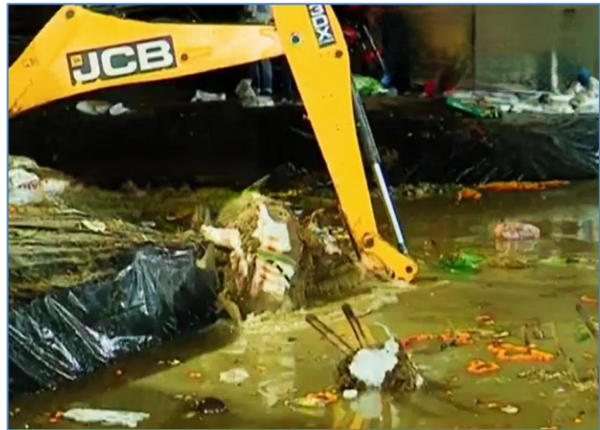
Fig. 7 Removal of Immersion left overs using JCB machine
