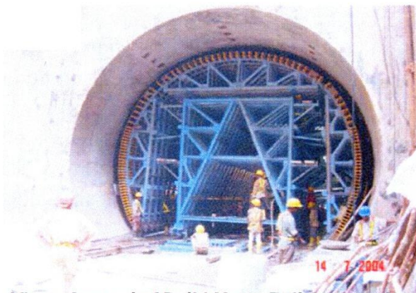
View of tunnel of Delhi Metro Rail Corporation where fly ash has been used
