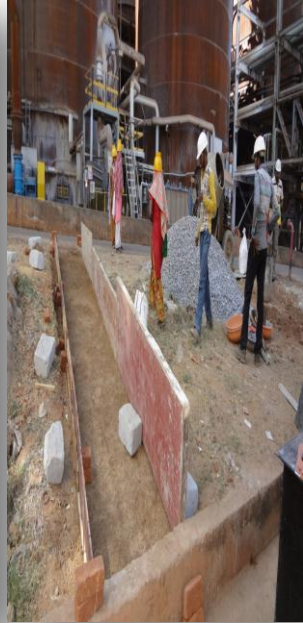
Construction Under prograss
