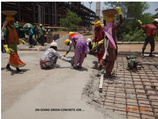
PCC POURING DURING GREEN CONCRETE MAKING
