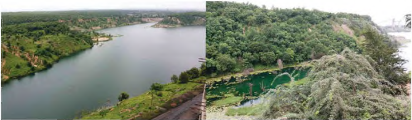
Fig-5.5 Water storage reservoirs in MCL area
